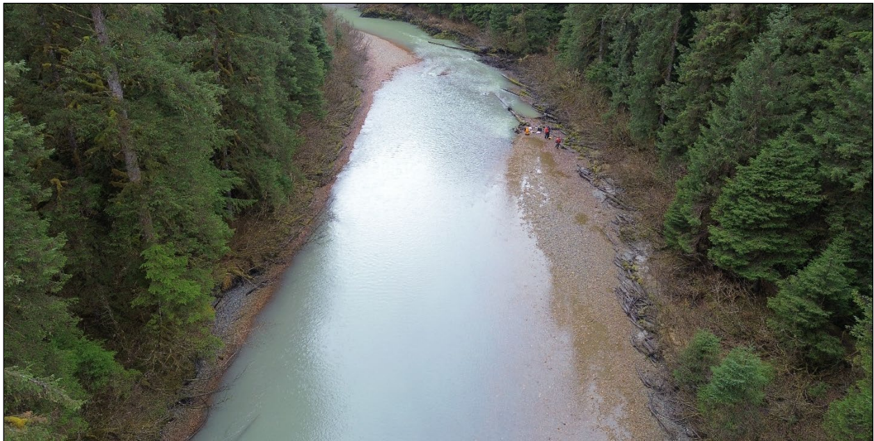
Figure 12.—Aerial view of the Lower Eagle River Site, 4/15/25.
